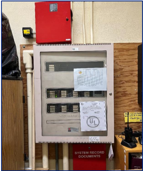
Existing Fire Alarm Control Panel
