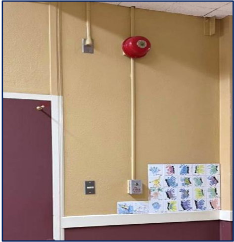
Existing Initiation & Notification Device
