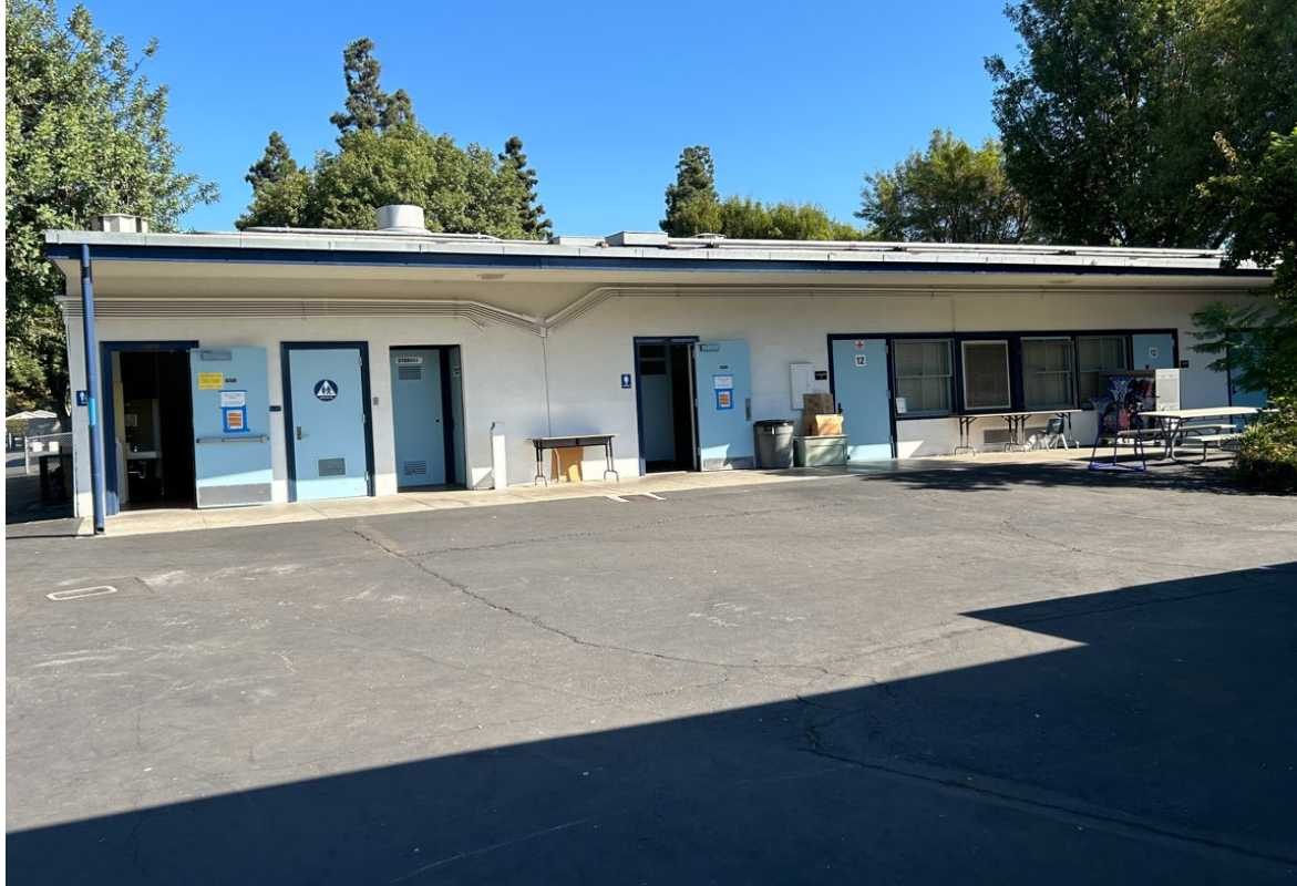
Cracked Asphalt in Playground
