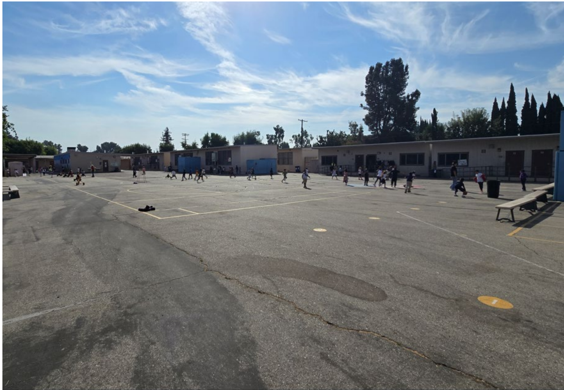
Cracked Asphalt in Playground
