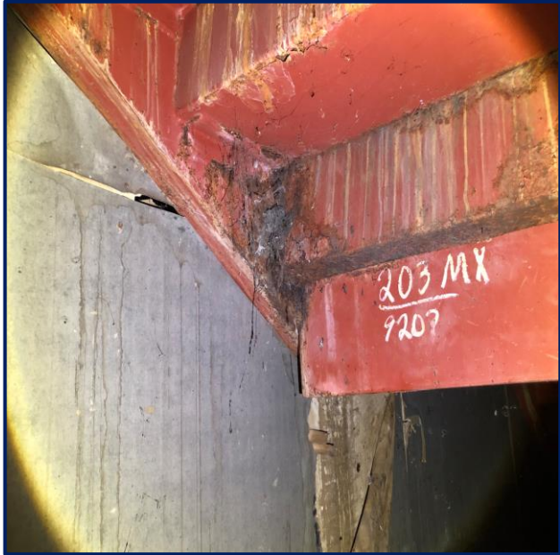
Deterioration Underneath Staircases
