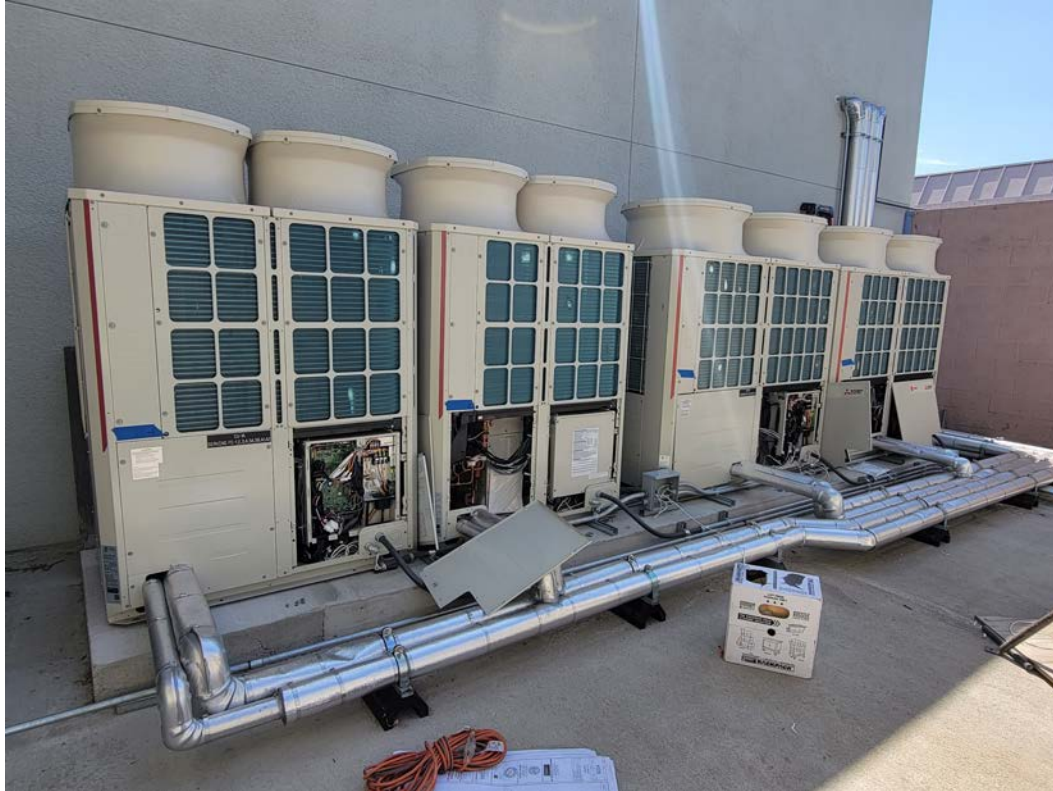
In Construction: Condenser Units Administration Building
