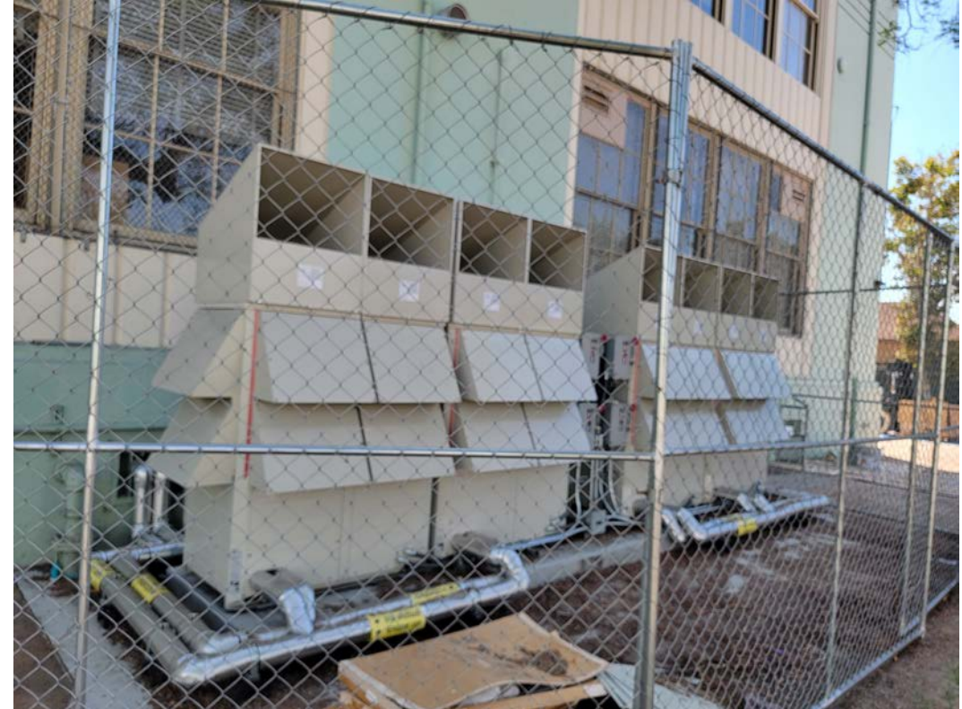
In Construction: Condenser Units Classroom Building
