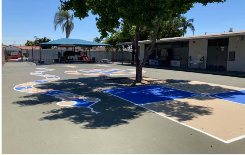
Completed: Solar Reflective Coating
