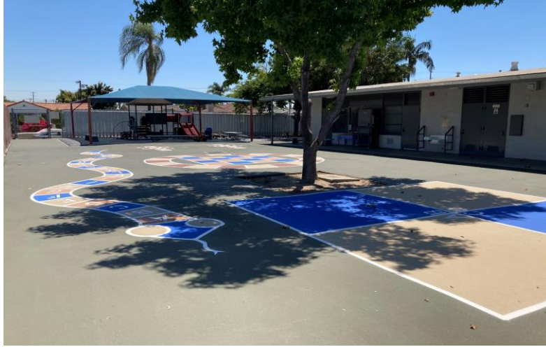
Completed: Solar Reflective Coating
