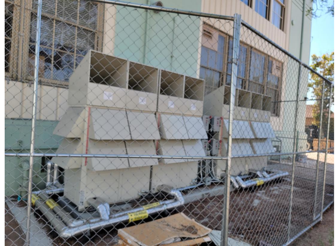
In Construction: Condenser Units Classroom Building
