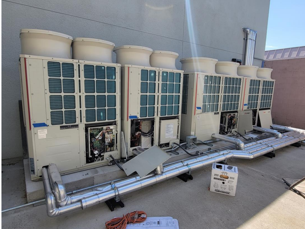
In Construction: Condenser Units Administration Building
