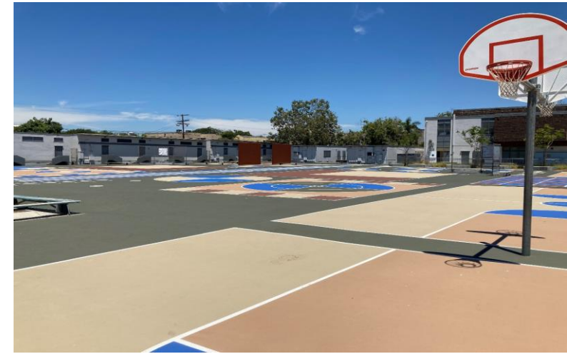
Completed: Solar Reflective Coating (East)
