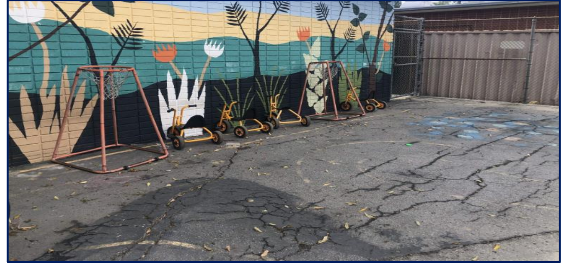
Deteriorated Asphalt
