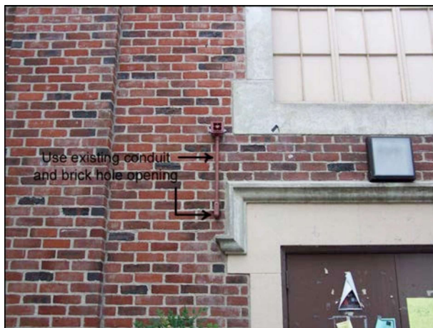
Figures 52. and 53. Re-use existing conduit connections and wall penetrations wherever possible. Source: ICF Jones & Stokes for LAUSD, 19 December 2008, "John Marshall High School Historical Resources CEQA Analysis for Fire Alarm System Upgrade Project."
