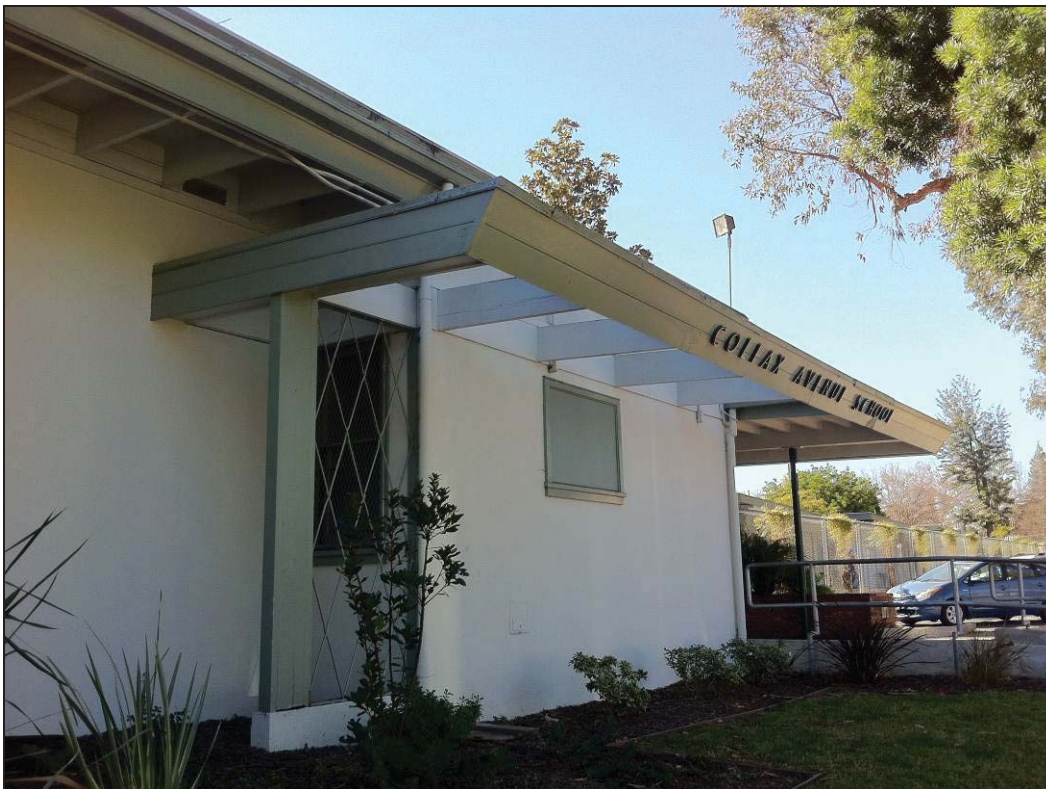
Colfax Avenue Elementary School, detail, Administration Building. Eaves extend to form an open grid around the entrance wing. Northeast perspective. Source: Sapphos Environmental, Inc., 21 January 2014.
