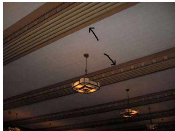
Figures 44. and 45. In this assembly hall, ducts and vents were placed and installed as unobtrusively as possible to avoid adverse impacts to many important character-defining interior features. Source: ICF Jones & Stokes, 13 July 2009, "Venice High School HVAC Project CEQA Analysis."
