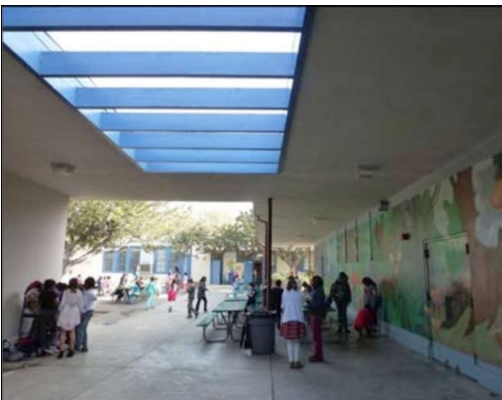
Figures 15. and 16. Mid-Century Modern roof treatments: flat roof with no eaves combined with cantilevered projections, Fernangeles Elementary School (left) and roof cut-out/skylight at Castle Heights Elementary School (1951, right). Source: LAUSD, 2014.
