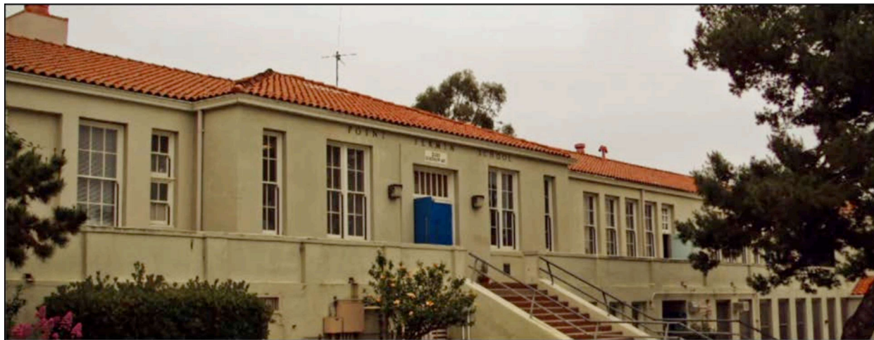
Figure 17. Shallow closed eaves and hipped-and-gable roof, clad in clay tiles, Point Fermin Elementary School, Administration Building (1917–1925; remodeled 1936). Source: LAUSD, 2010.
