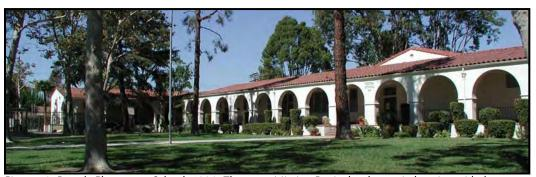
Figure 12. Reseda Elementary School, 1936. The spare Mission Revival style was in keeping with the post-Field Act requirement for one-story massing and the post-Long Beach Earthquake trend to design in the "traditional Southern Californian" mode. Source: LAUSD.
