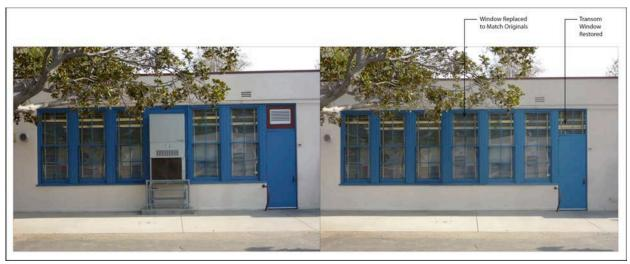
Figure 39. Removing inoperable HVAC units and returning windows to original use can greatly enhance a historic school building. Image on left shows HVAC unit currently in place at Castle Heights Elementary School; image on right simulates the building's appearance following replacement of HVAC unit. Source: Architectural Resources Group, 2014.
