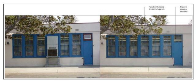
Figures 46. and 47. Where possible, removing inoperable HVAC units and restoring windows to match originals enhances the appearance of historically significant LAUSD buildings. Source: LAUSD and Architectural Resources Group, 2014.
