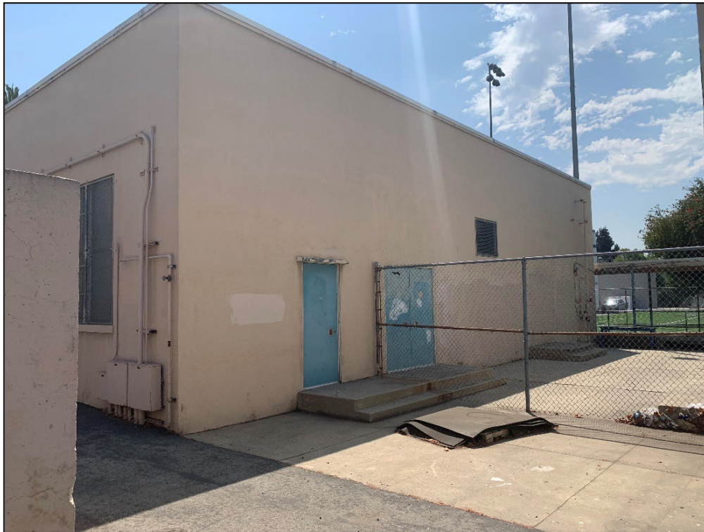
Figure 75. Southwest façade of Shop No. 2, view toward the east.
