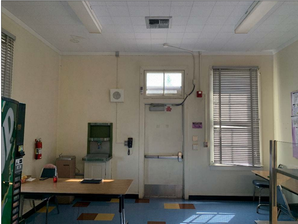
Figure 66. Two-light transom and Moderne-style water station in Faculty Dining Room in Cafeteria.
