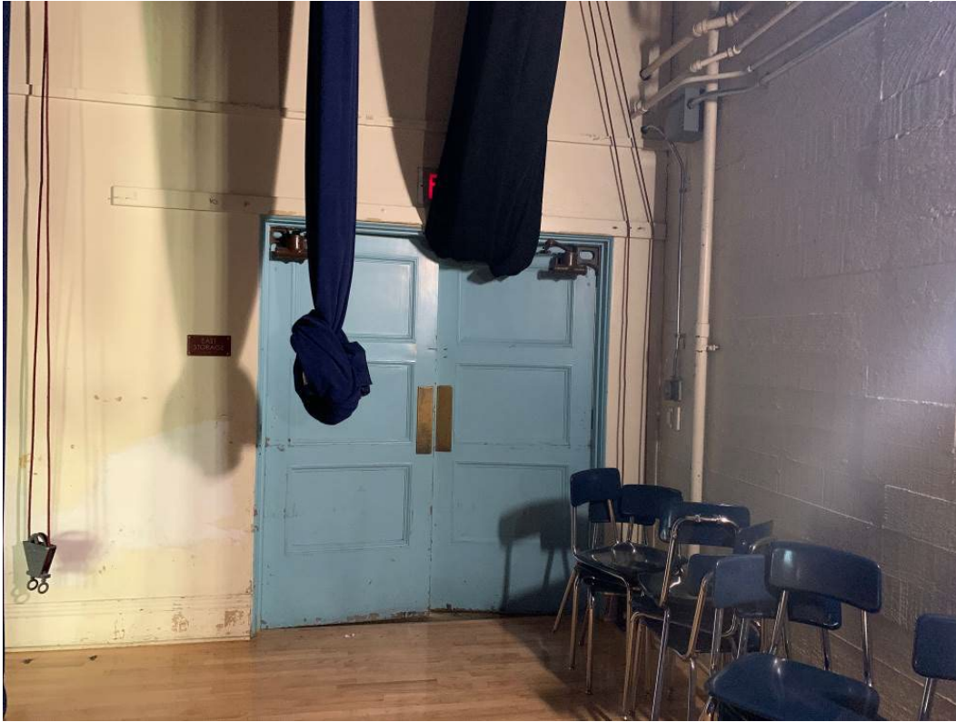
Figure 48. Wood flooring on stage and backstage area and two-panel wood doors.
