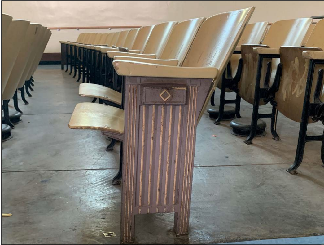
Figure 44. Detail of cast-iron and molded plywood foldable seating in Auditorium.
