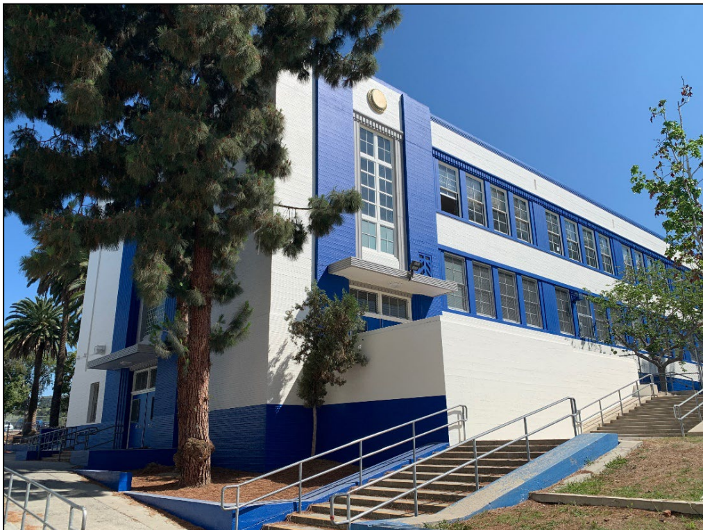
Figure 14. Southwest and southeast façades of the Administration building, view toward the north.
