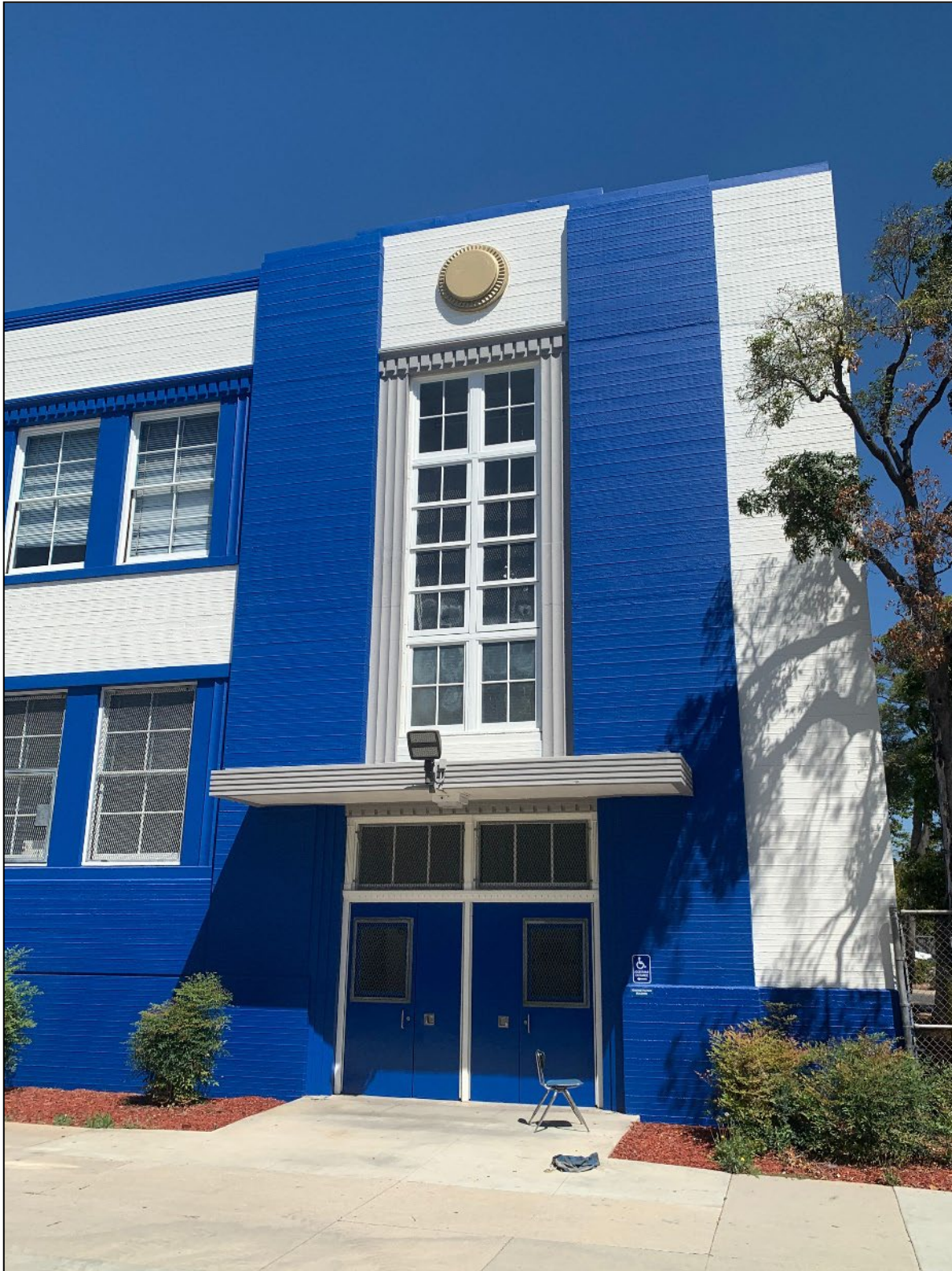
Figure 12. Secondary entrance at southeast façade, showing horizontal board-formed concrete texture on exterior walls.
