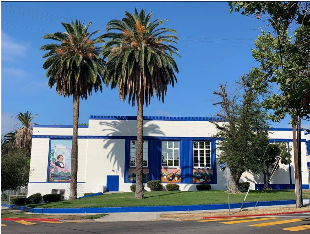
Figure 34. Northeast façade of Auditorium. Shows crested stringcourse at top of parapet, dentil stringcourse above windows, and multi-light wood windows, view toward the southwest.
