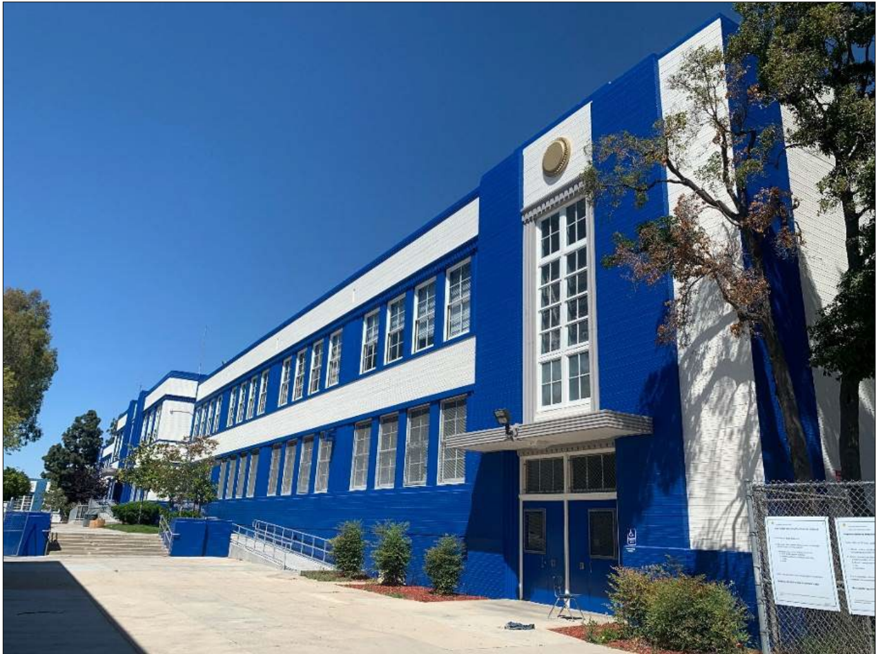
Figure 11. Southeast façade of the Administration building. Shows horizontal stringcourses and configuration of secondary entrances, with flat canopy, vertically oriented window, and plaster medallion.
