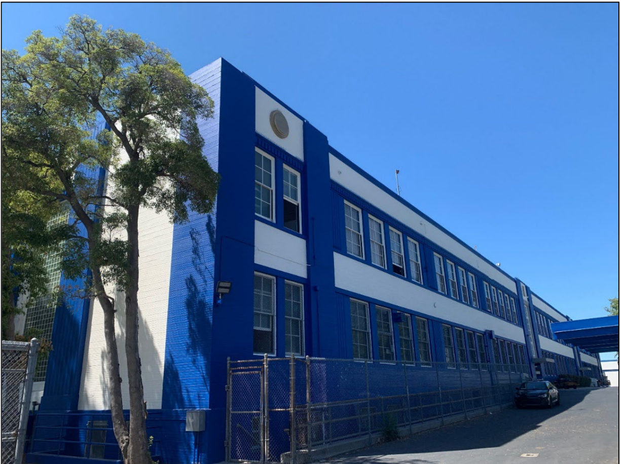
Figure 15. Northwest façade, view toward the south.
