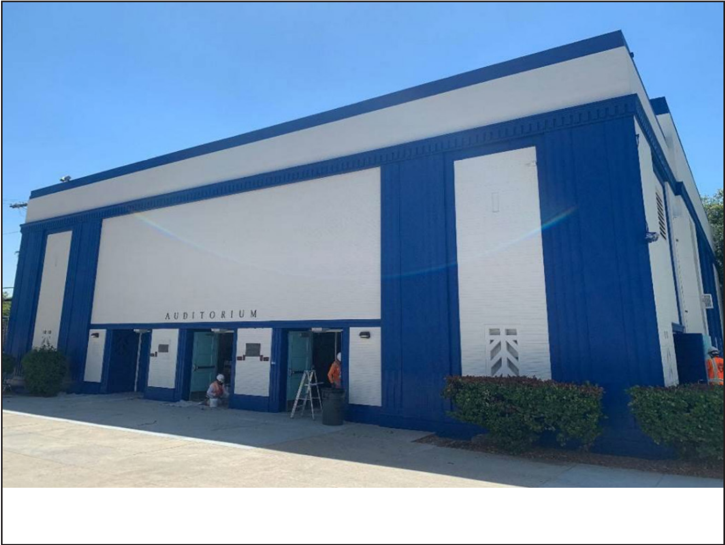
PHOTO 6 Auditorium Primary (northwest) facade source LAUSD Final HRER by ASM
