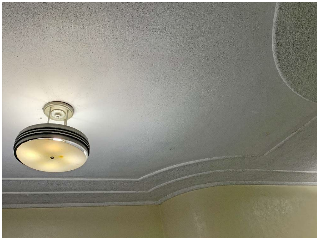
Figure 41. Detail of chandelier and curvilinear ceiling motif in Auditorium lobby.
