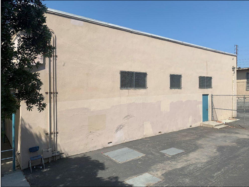
Figure 73. Northeast façade of Shop No. 2, view toward the west.
