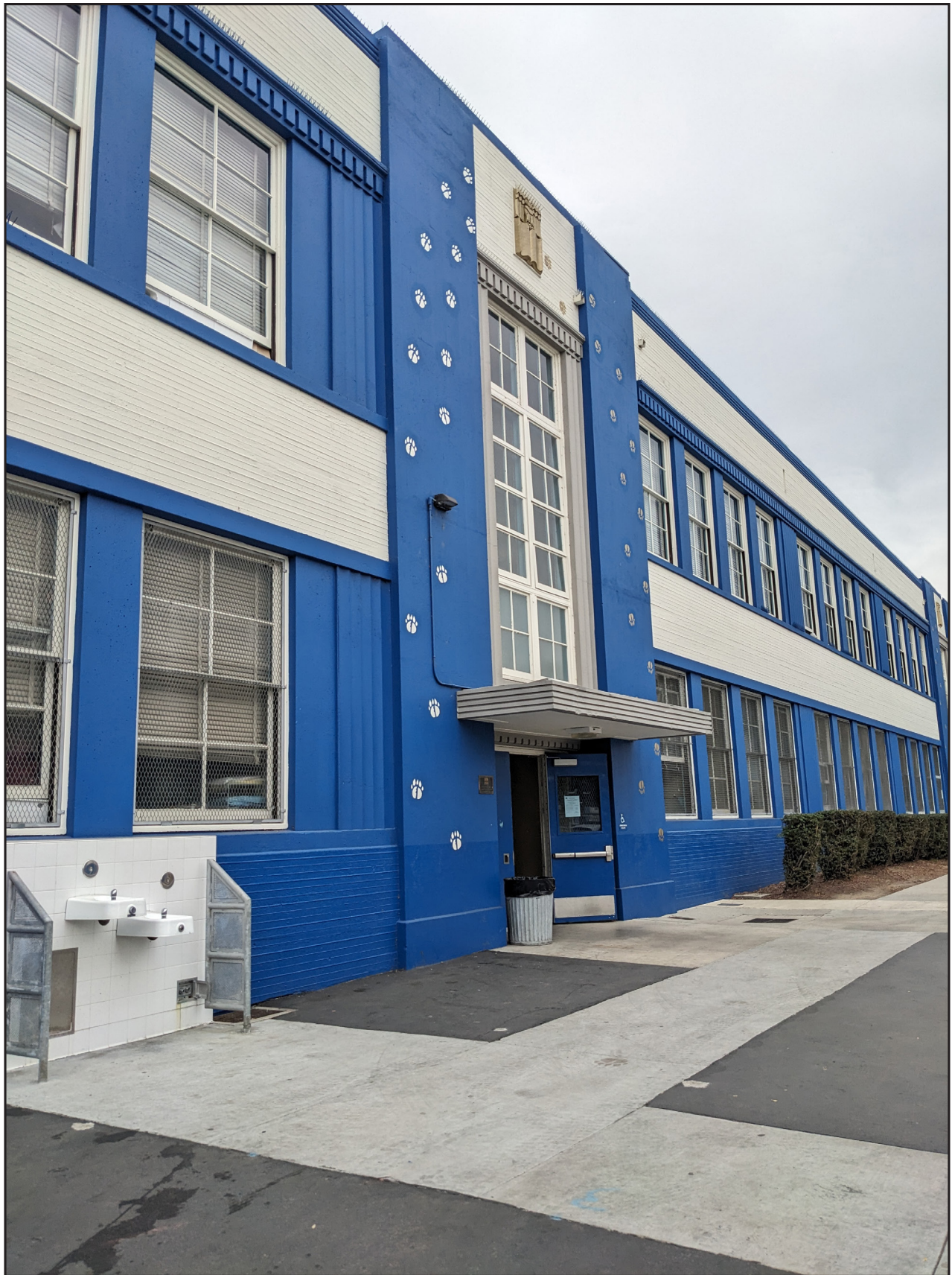
PHOTO 1 Admin Northwest Facade IMS
