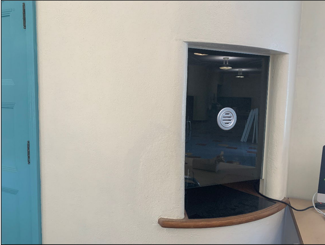
Figure 40. Rounded wall and ticket booth in foyer, view toward the northwest.
