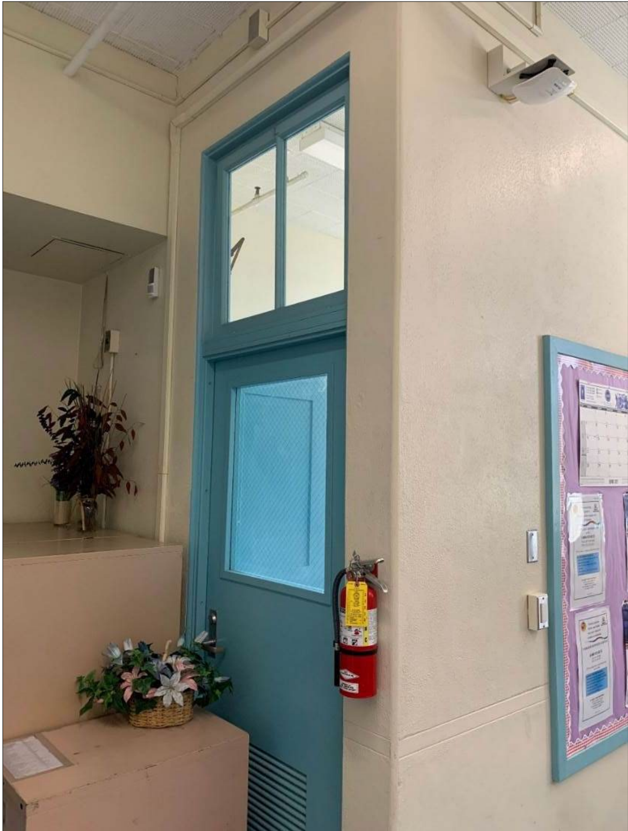
Figure 23. Two-light transom in Administration Building.
