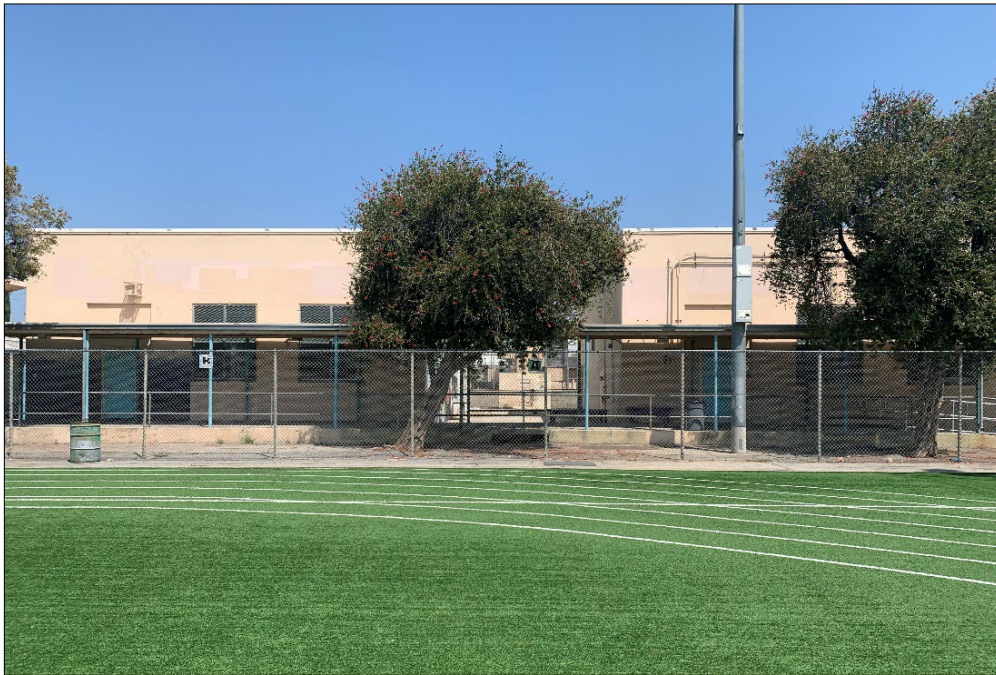
Figure 68. Southeast façades of shops, view toward the northwest.
