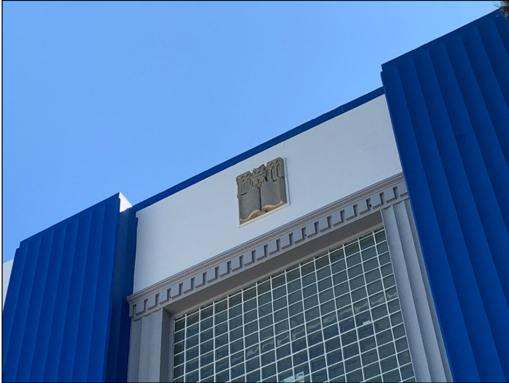
Figure 13. Detail of plaster medallion in form of an open book with owl above on the southwest façade, view toward the northeast.
