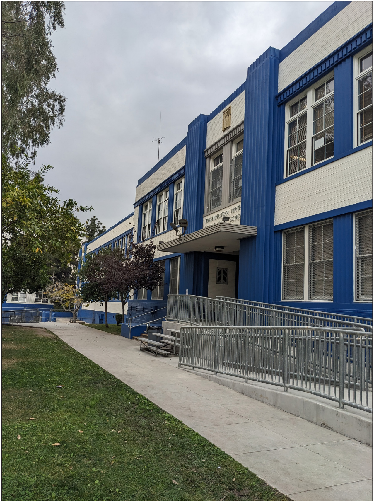
PHOTO 2 Admin Southeast (Primary) Facade Admin IMS
