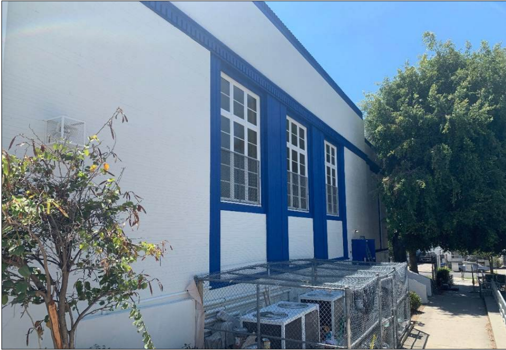
Figure 35. Southwest façade of Auditorium. Shows window configurations identical to northeast façade.
