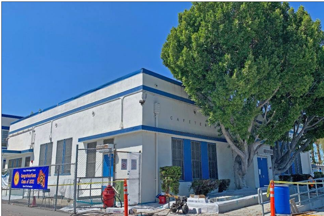
Figure 62. Stringcourse, canopies, and sunshades with horizontal details on Cafeteria.
