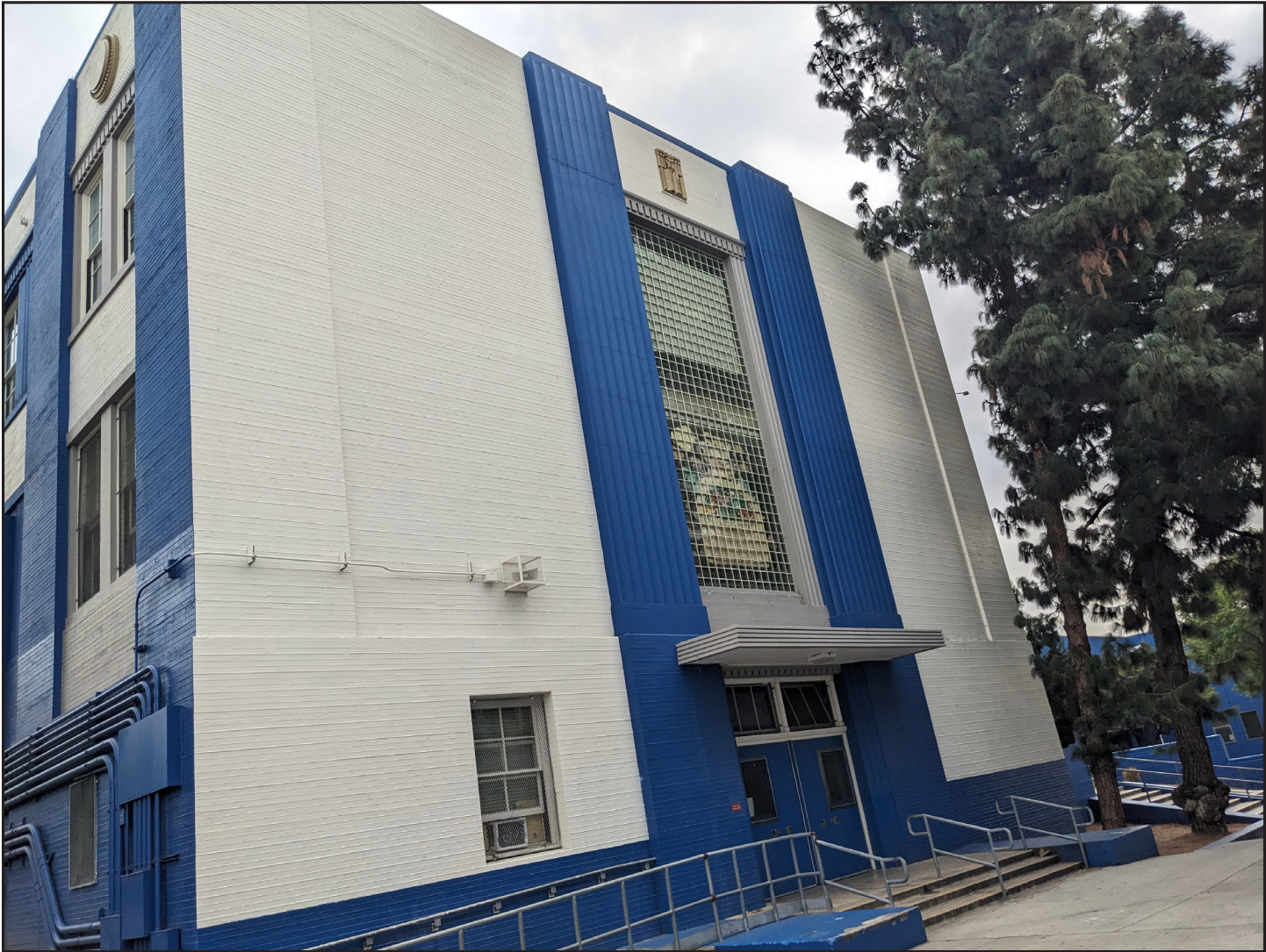
PHOTO 3 Admin Southwest Facade Admin Bldg IMS
