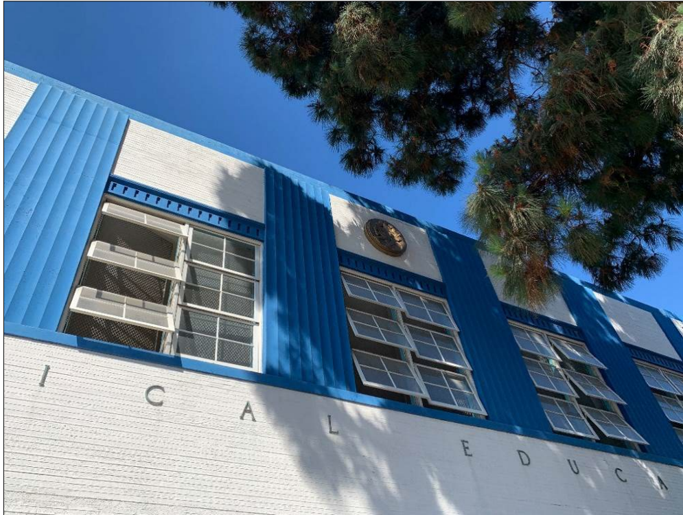
Figure 52. Detail of cut-out letters and awning-type windows at northeast façade of Physical Education Building.
