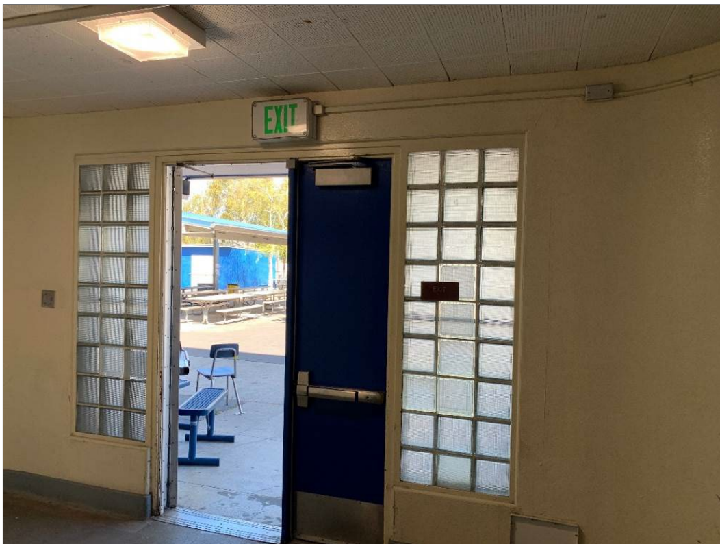
Figure 21. Glass blocks flanking ground-floor entrance.
