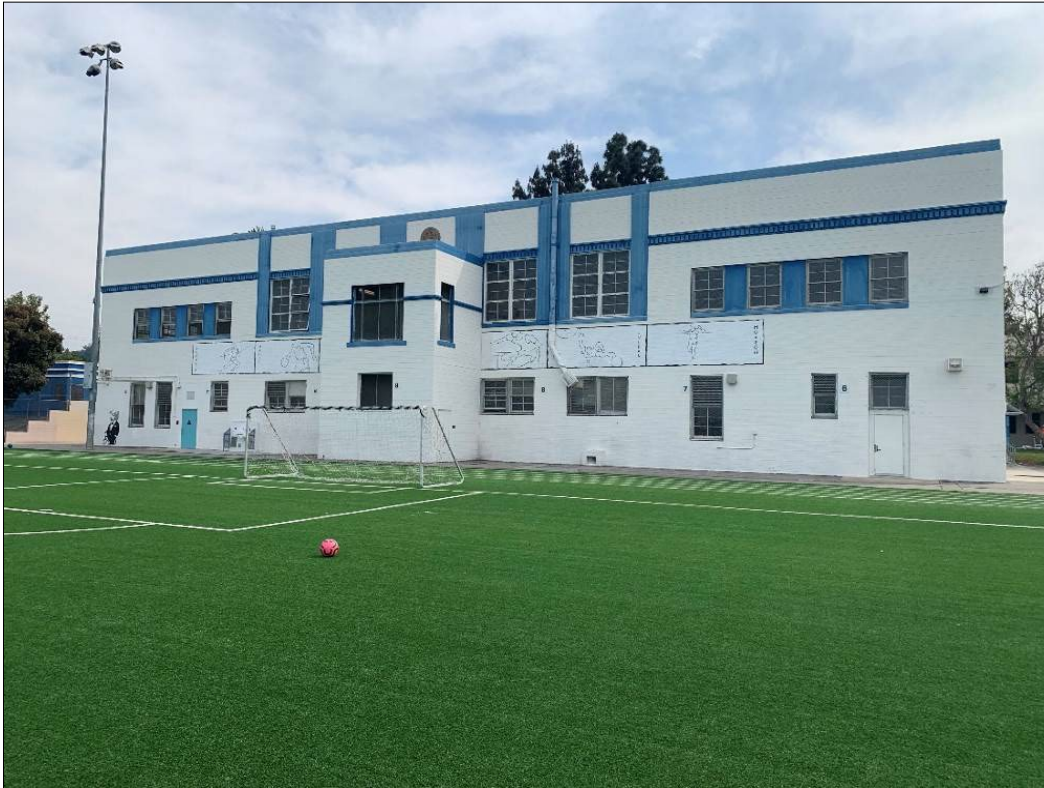
Figure 53. Window configurations at southwest façade mirror those at primary façade.
