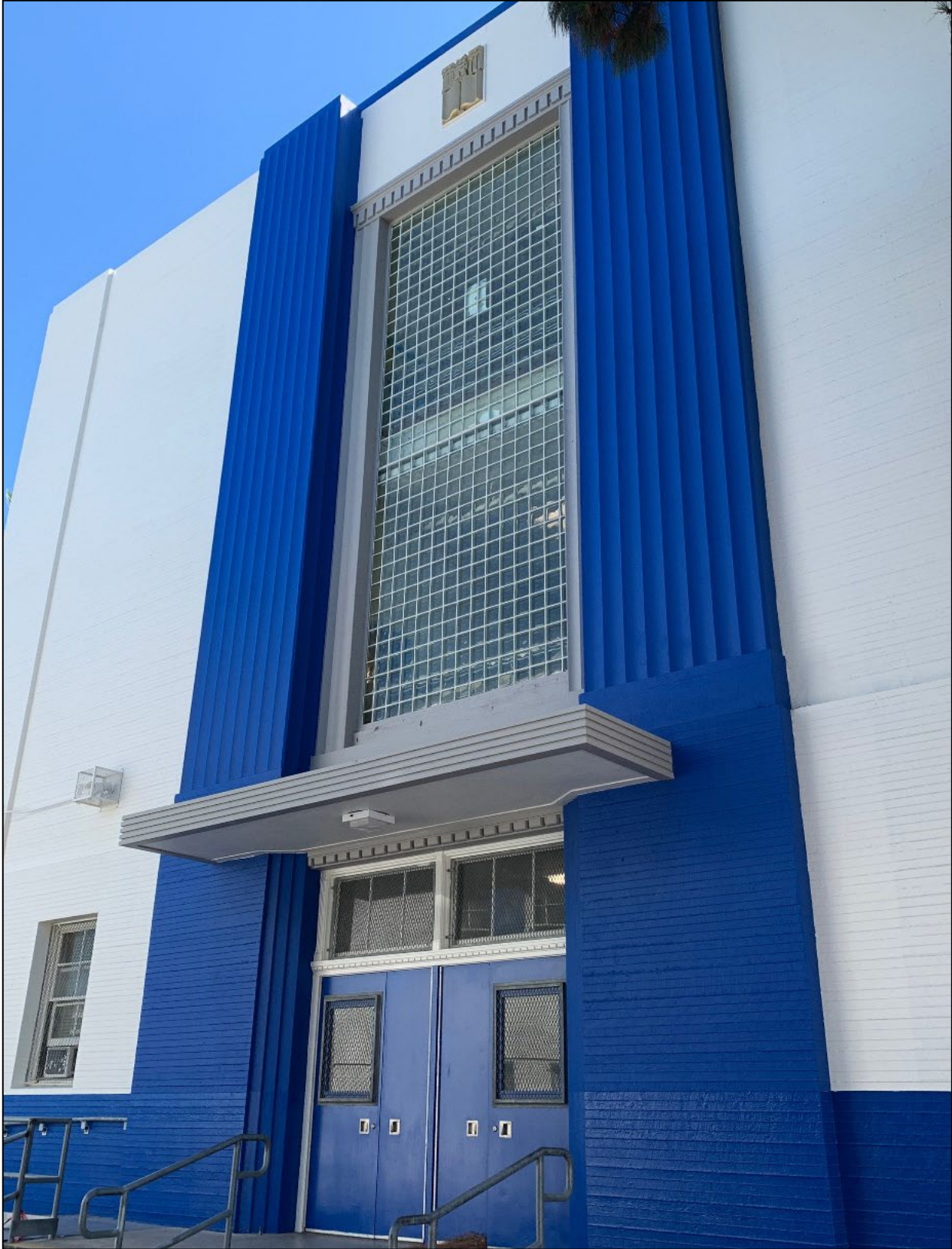
Figure 18. Southwest façade of the Administration building, view toward the northeast.
