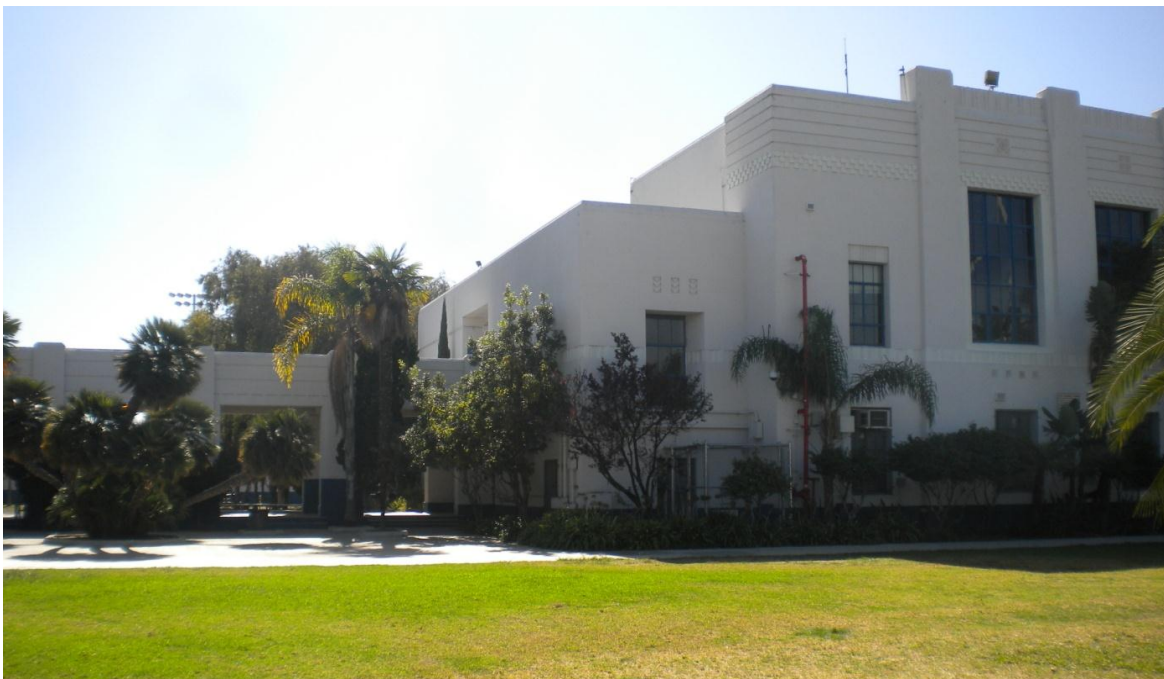
View of the Historic Administration Building and Bridge #2 located along Venice Boulevard.
