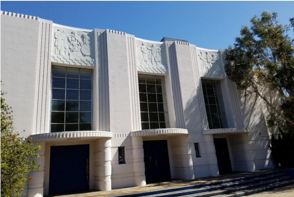
View of the Auditorium (Assembly Hall) main entrance (exterior) along Venice.
