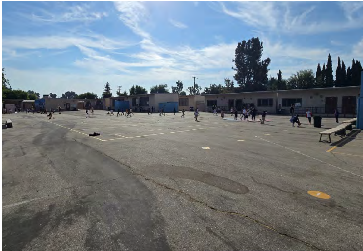
Cracked Asphalt in Playground
