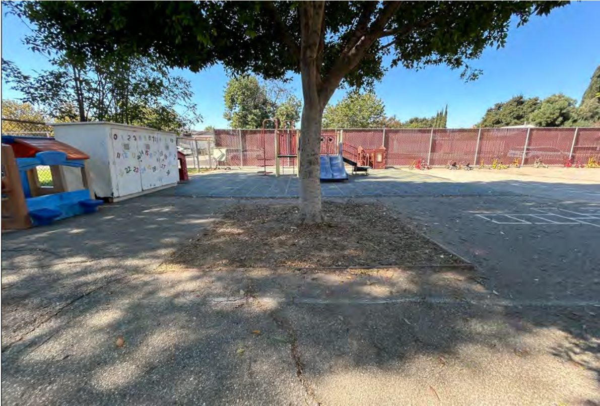
Cracked Asphalt in Playground
