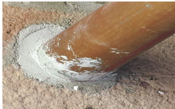
The opening around this pipe has been sealed with concrete to keep pests out.
