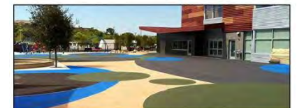
COLOR COAT SURFACE ON ASPHALT
