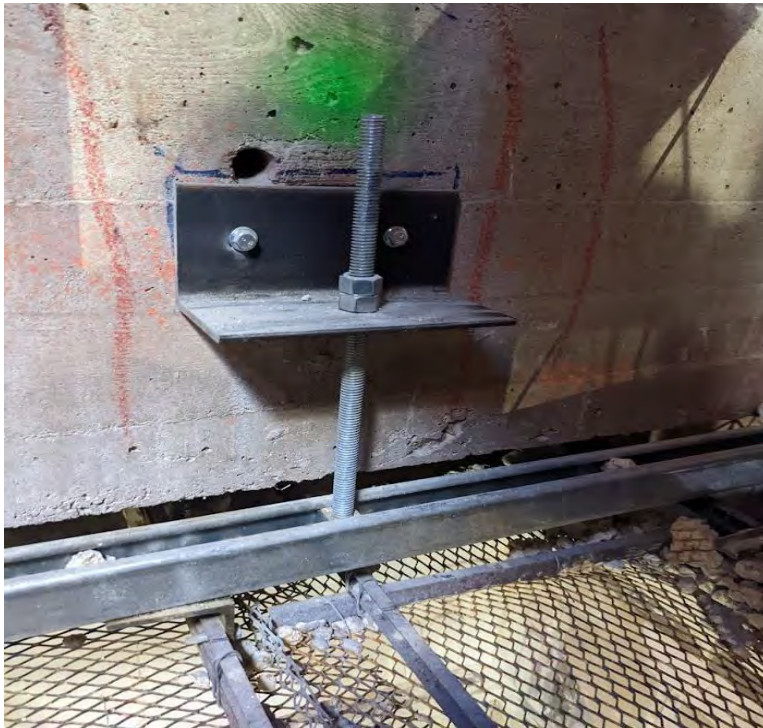
Ceiling system framing secured to walls
