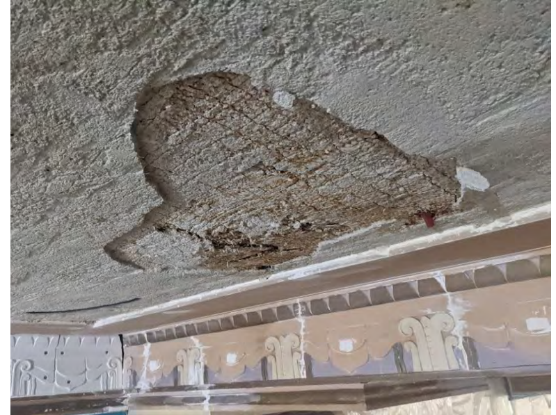
Removal of prior plaster repair
