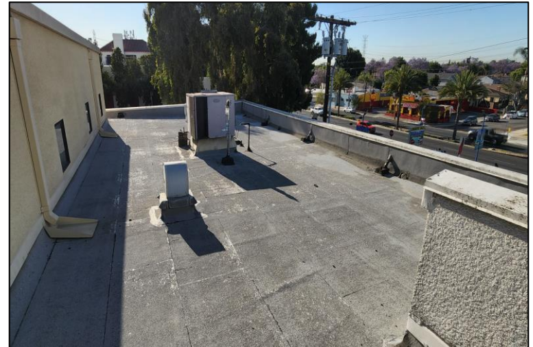
Deteriorated Roofing
