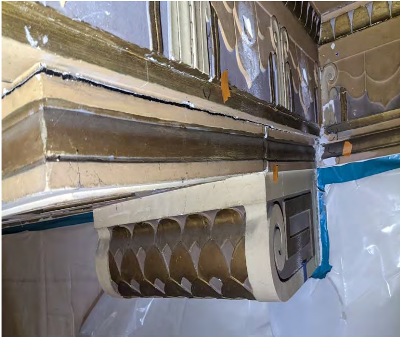
Corbels separating from the ceiling
