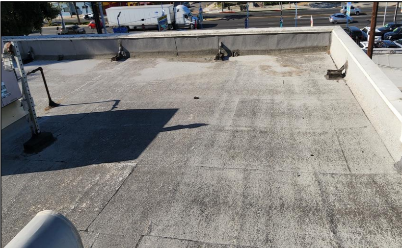
Deteriorated Roofing
