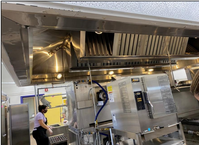
Kitchen Hood without Fire Suppression System
