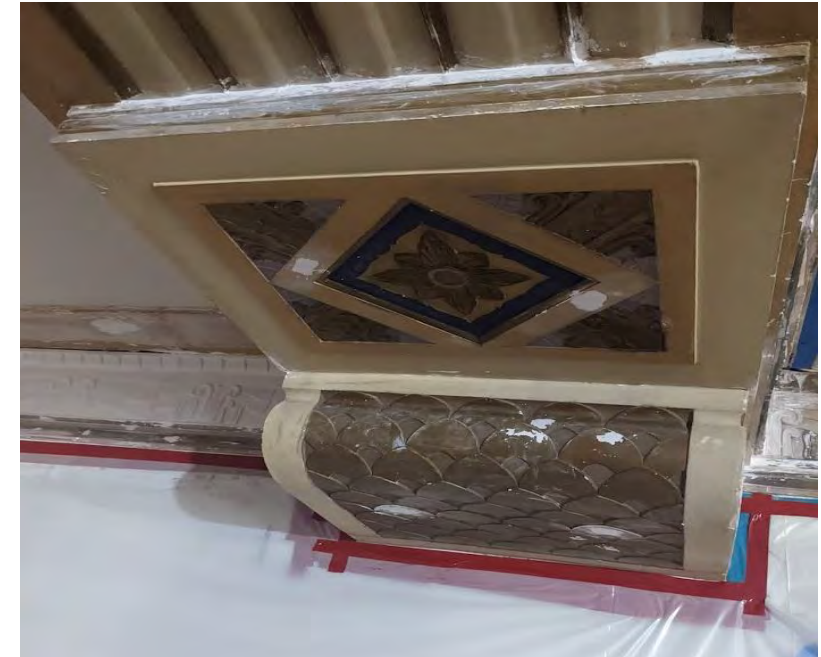
Corbel repair work (from below)
