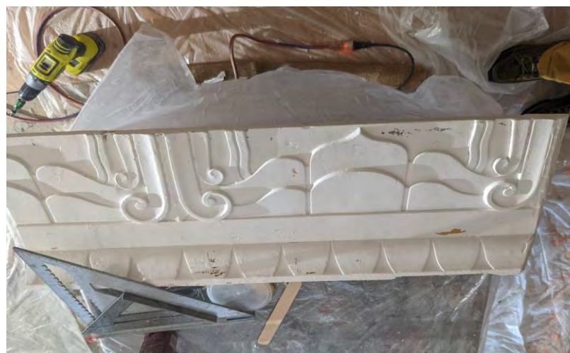
New panel from plaster cast
