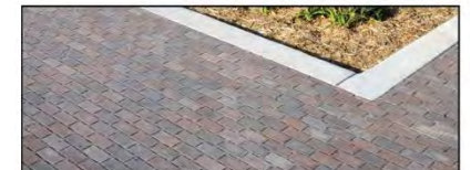
INTERLOCKING PAVERS
