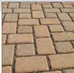
INTERLOCKING CONCRETE PAVERS
