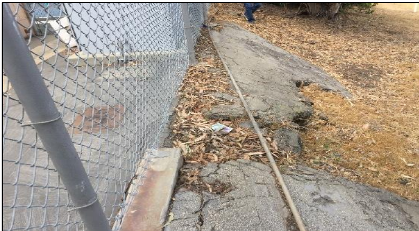
Deteriorated Asphalt at Slope
