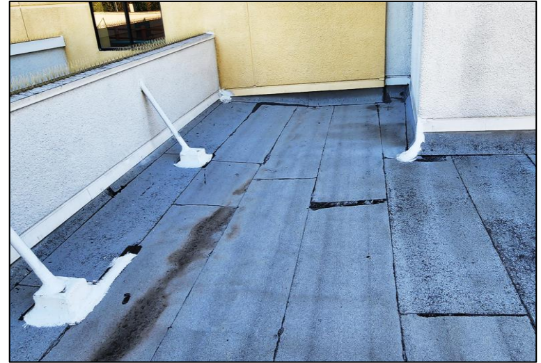
Deteriorated Roofing
