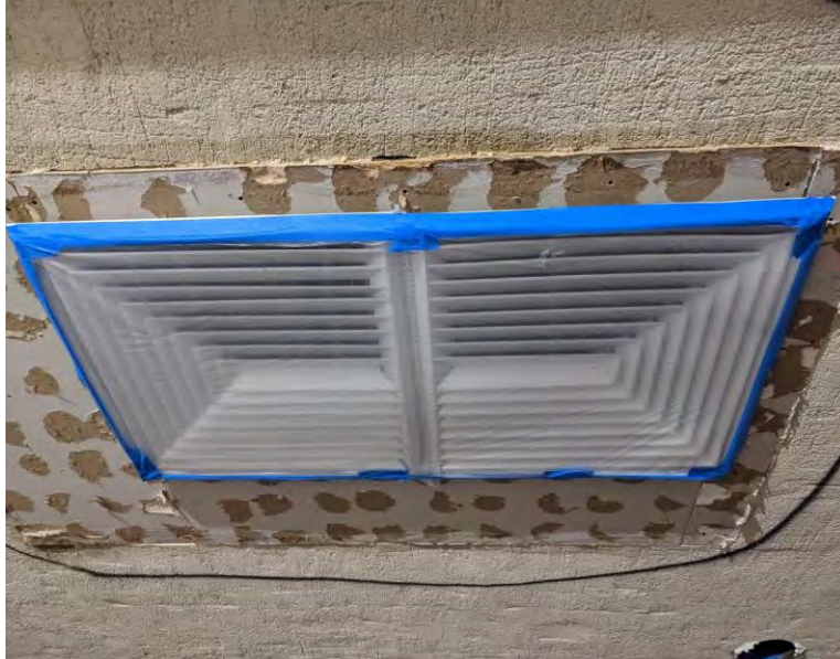
Removal of patched drywall
