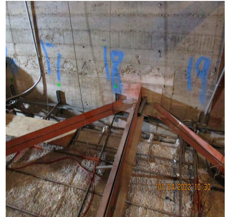
Seismic separation at wall
