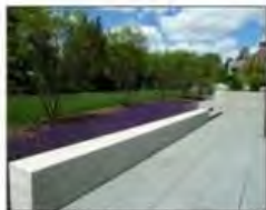
CONCRETE SEAT WALL
