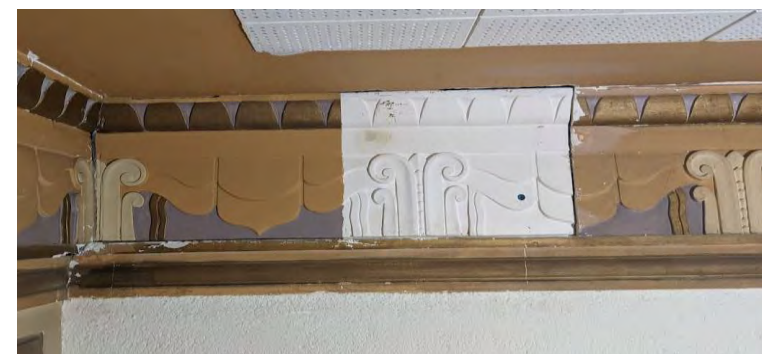
Installation of new panels
