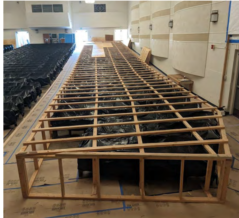
Building wooden enclosure around seats
