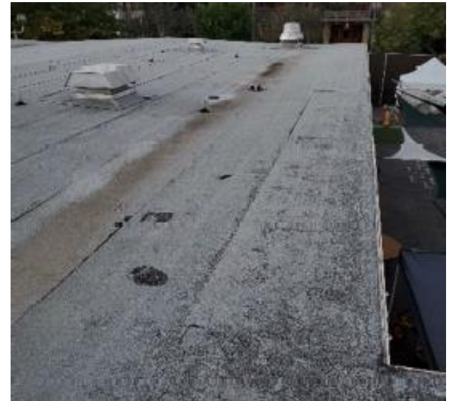
Deteriorated Roof
