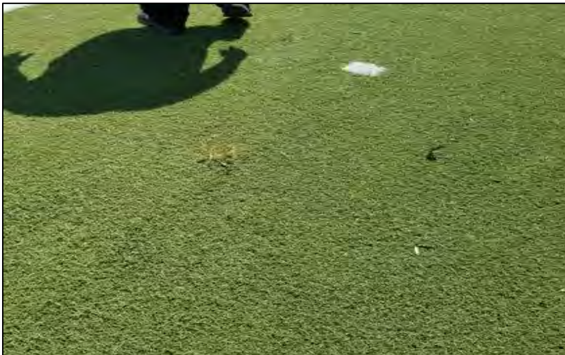
Melted Infill
