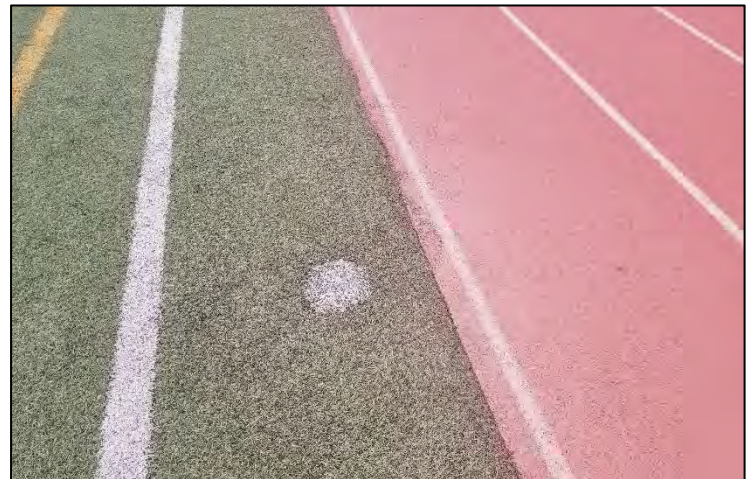
Deteriorated Synthetic Turf
