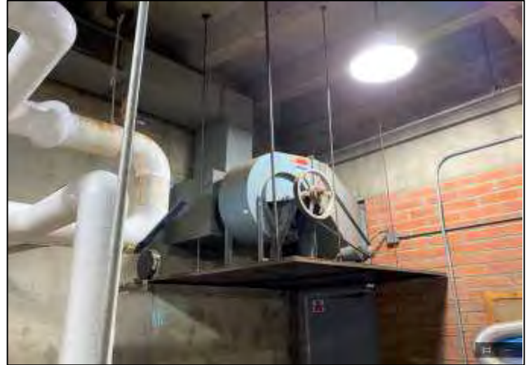
Suspended Utility Exhaust Fan
