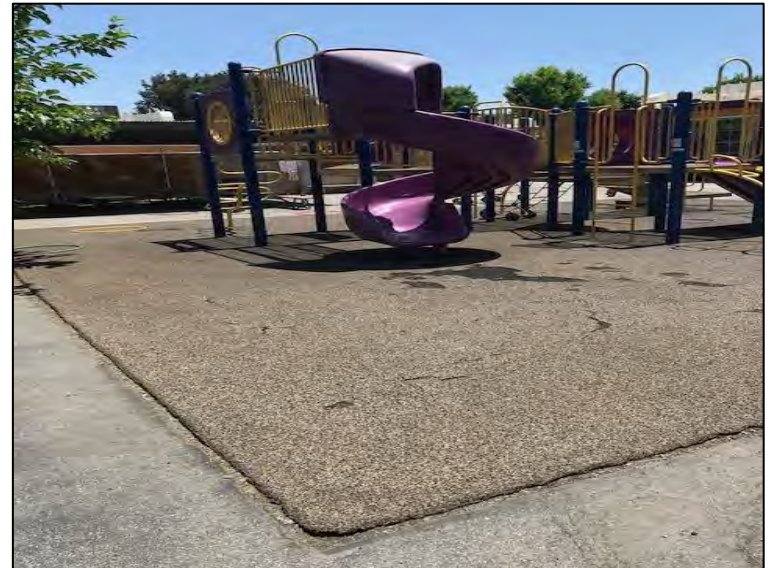
Deteriorated Playground Matting and Antiquated Equipment
