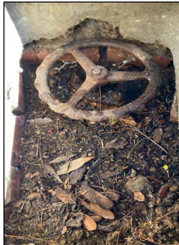
Deteriorated plumbing piping and shut off valves
