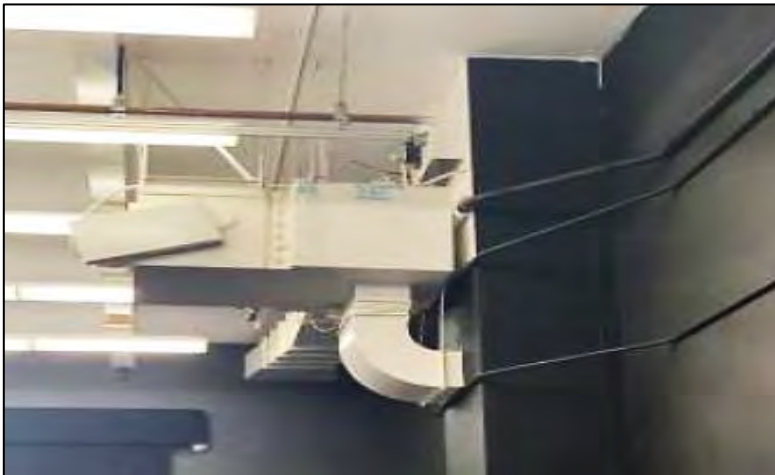
Suspended Heating & Ventilation Unit
