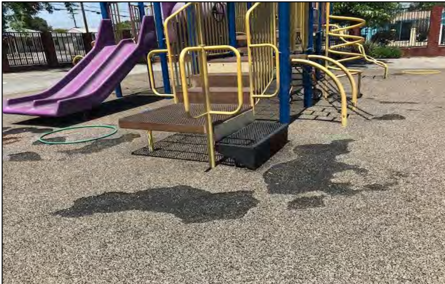
Deteriorated Playground Matting and Antiquated Equipment
