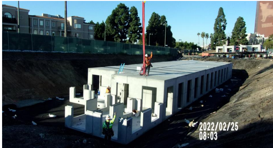
Stormwater Detention Tank
