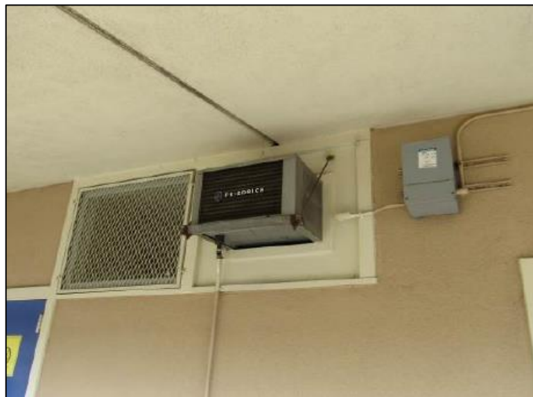
Typical Window Air Conditioning Unit
