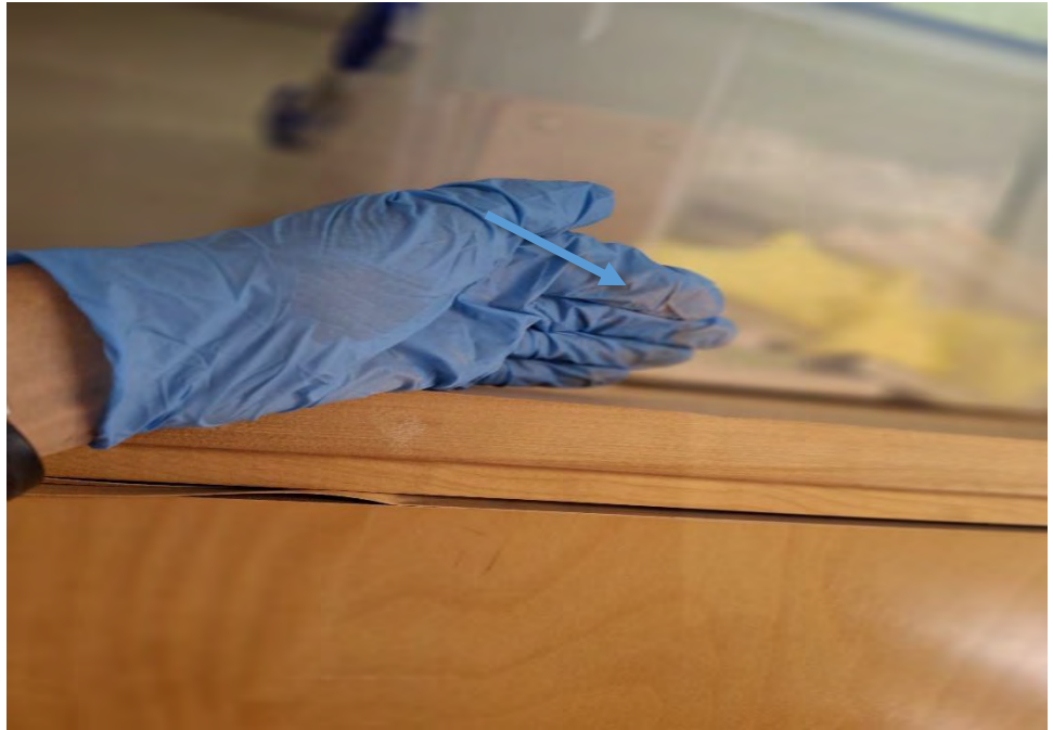
Photograph 4: View of DSA building Shelves. Smoke/ fire debris observed
