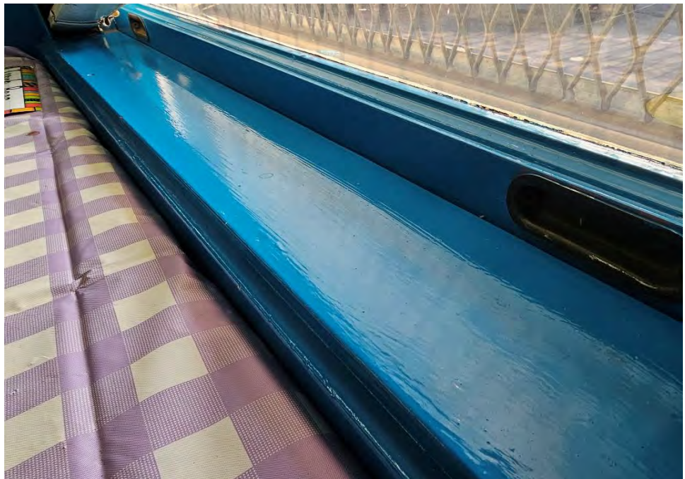
Photograph 12: View of Building C classroom 21 window sill. No smoke/fire debris observed.
