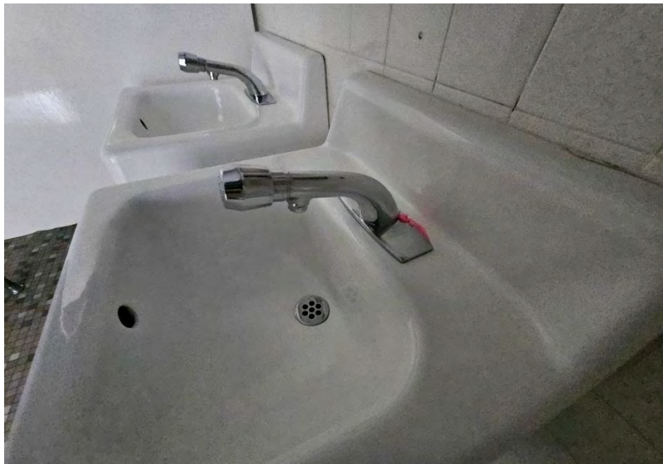
Photograph 14: View of Building C Boy's restroom sinks. No smoke/fire debris observed.
