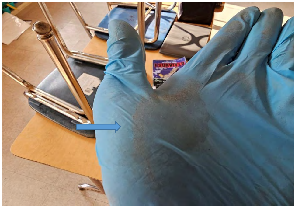
Photograph 20: View of Building AA-1138 Classroom 3 and 4 smoke/fire debris observed on the desks.
