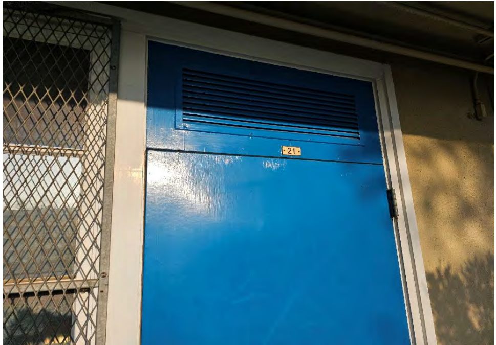
Photograph 11: View of Building C classroom 21.
