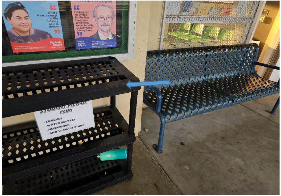
Photograph 5: View of the main office student lunch drop off shelf. Visible smoke/fire debris.
