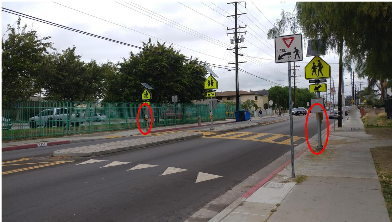
Although not under the direct control of LAUSD, control boxes strapped to the pole underneath RRFB signs, are mounted over the sidewalk with low vertical clearance, and therefore may pose an obstruction.
