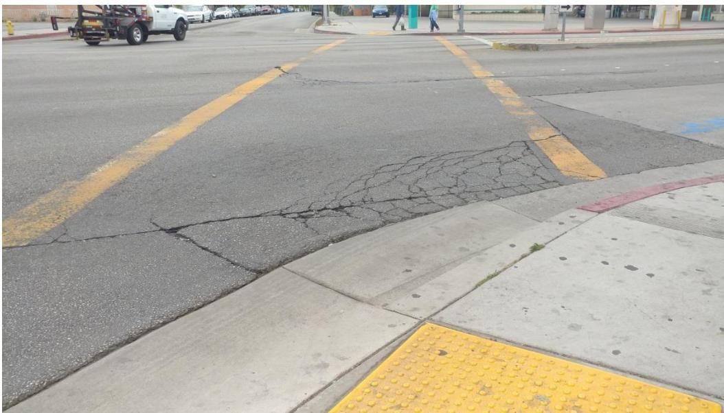
Crossing pavement markings are worn and cracked on the intersection of Clara Street and Atlantic Avenue.
