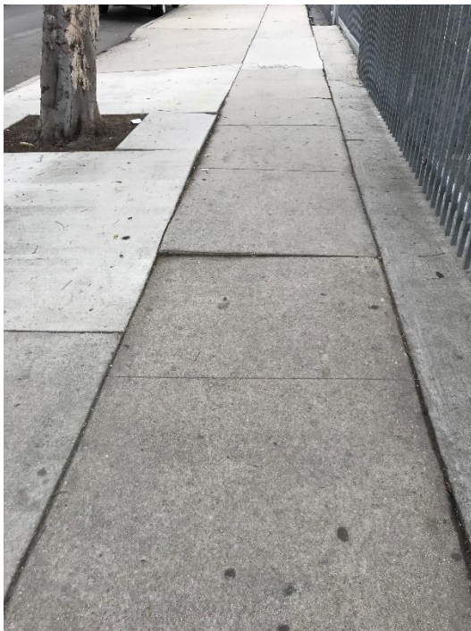
Tree roots lifting sidewalk can cause a difficult walking environment on East 78th Street
