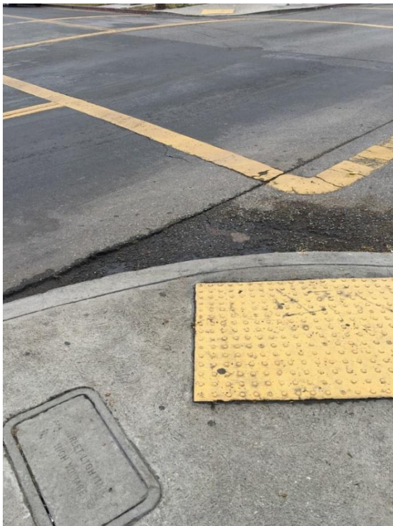
Curb ramp in the northeast corner of the intersection East 79th Street and McKinley Avenue has possible ponding, degraded pavement, and vertical grade differences over one-half inch
