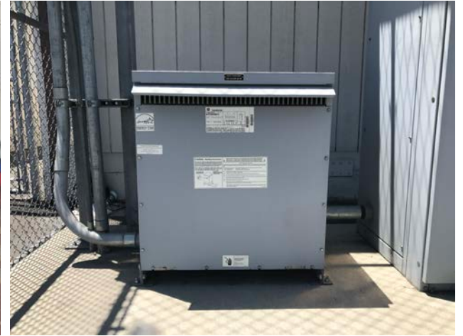
Photograph 9. View of one of three onsite pad-mounted transformers.
