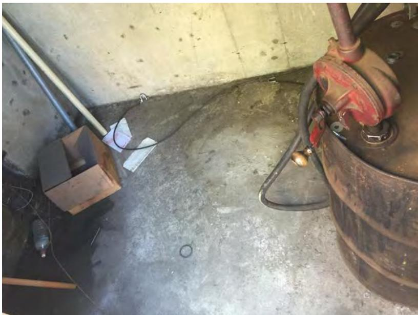
**Photo 14:** 55-gallon drum storing gasoline and hydrocarbon staining/spill, in the flammable materials storage building, located southeast of Building No. 9 (Shop Building).
