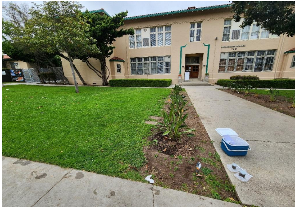
Photograph 1: Exterior of Brentwood Science Magnet Administration Building.
