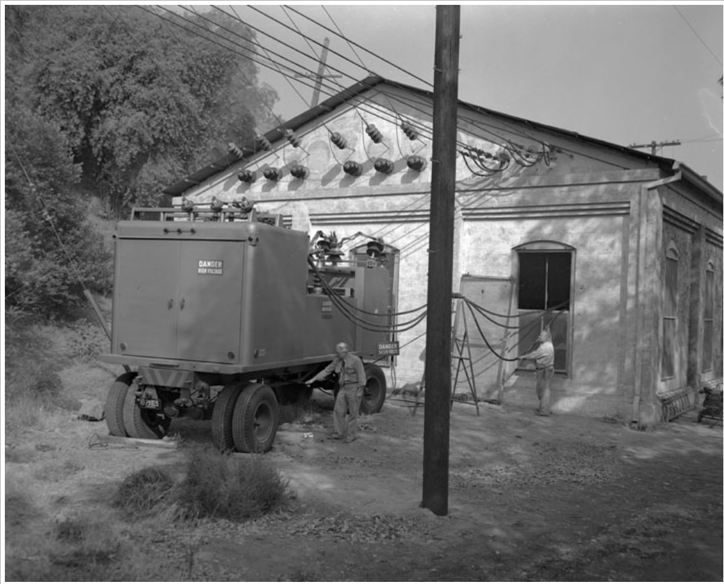
(1952)* - View showing the portable distributing station being used as a sub-station.
