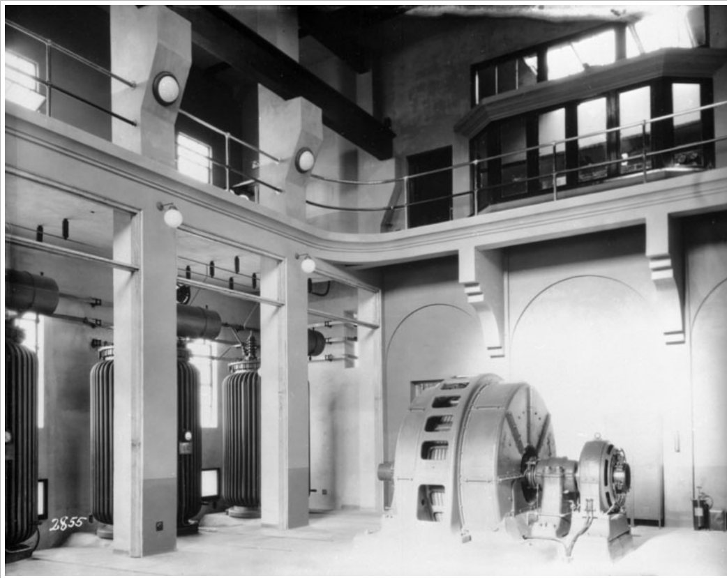
(ca. 1920s)* - Interior view of DS-3 showing station transformers (left) synchronous condenser (right).
