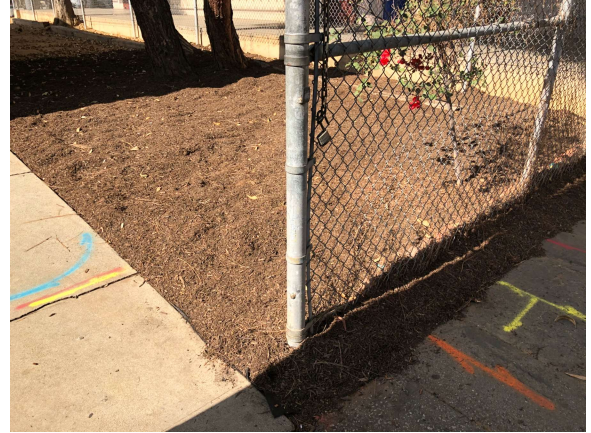
Unpaved portion of AOC 6 after placement of geotextile and mulch 11/12/2019 11:44
