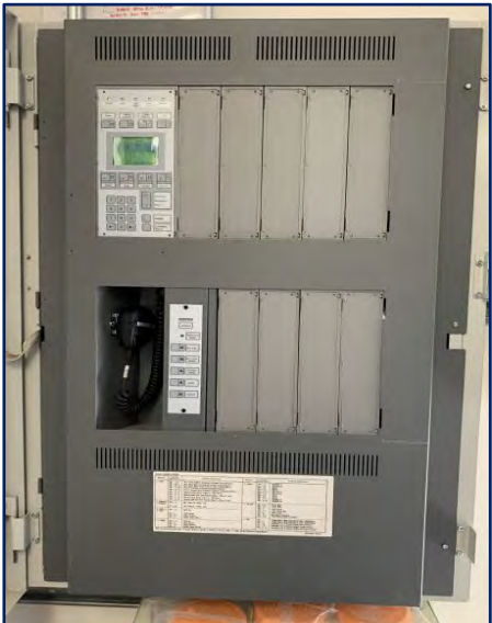
Example of New Fire Alarm Control Panel
