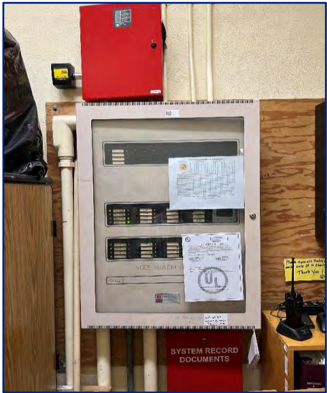
Existing Fire Alarm Control Panel
