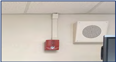
Example of New Smoke Detector Initiating Device & Speaker-Strobe Notification Device
