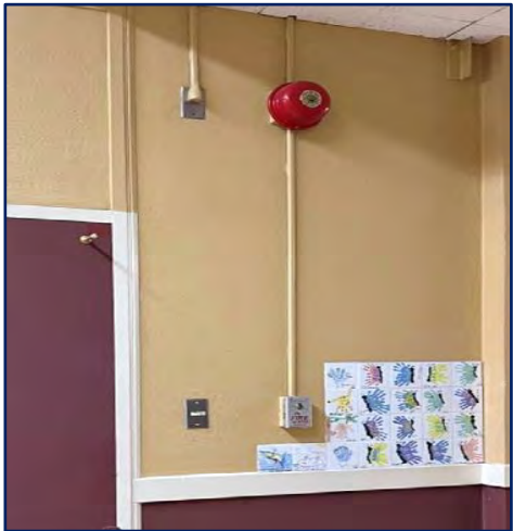
Existing Initiation & Notification Device
